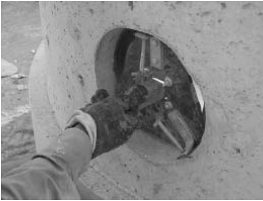
#1 ASSEMBLY STARTS WITH CENTERING TRIANGLE IN LOW HOLE
