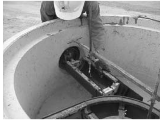
#4 POSITION ANTI FLOTATION BAR AND ADDITIONAL CHANNEL
