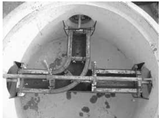
#6 COMPLETED THREE-WAY ASSEMBLY READY TO POUR
