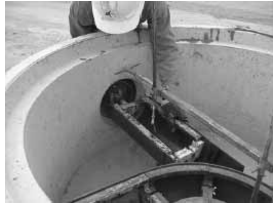
#4 POSITION ANTI FLOTATION BAR AND ADDITIONAL CHANNEL
