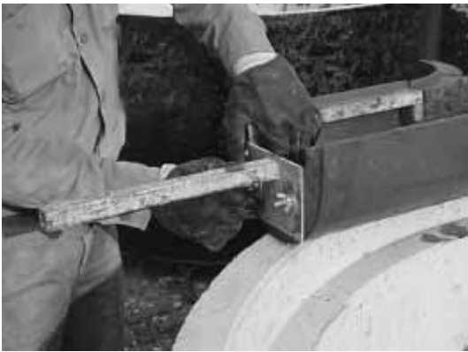
#2 ASSEMBLE SMALLEST ANGLE WITH CENTERING ADAPTOR
