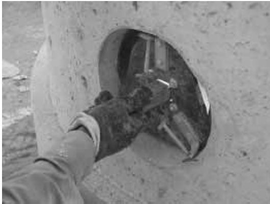
#1 ASSEMBLY STARTS WITH CENTERING TRIANGLE IN LOW HOLE
