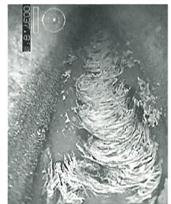
Gasoline can be seen mixing with water in the storm sewer.
