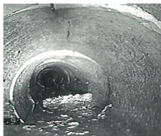
R & R Visual was able to determine where leaked fuel infiltrated a stormwater collection system with a Pearpoint video inspection system.
