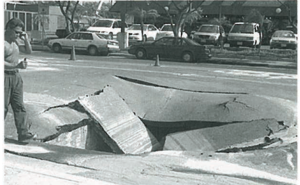
What a safety hazard! What do you think it will cost to repair this major intersection in Honolulu, Hawaii where a roadway collapsed around a storm drain?
