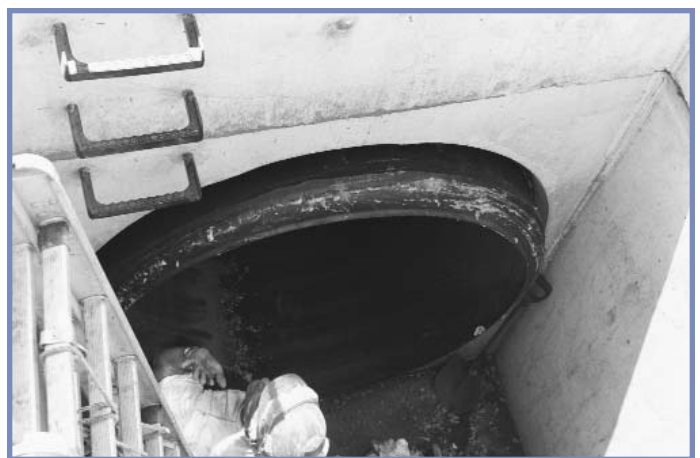
COMPLETED WATERTIGHT CONNECTION
