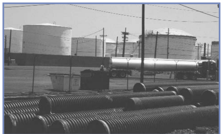
THE JOB SITE
