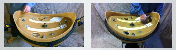
Place the inside mandrel half on top and hand-tighten nuts and bolts. Make sure the waterstop is perpendicular to the outside wall of the mandrel. Then look through all observation holes to be sure the nose of the connector is still up against the offset. Tighten nuts with wrench. Re-check waterstop and observation holes.
