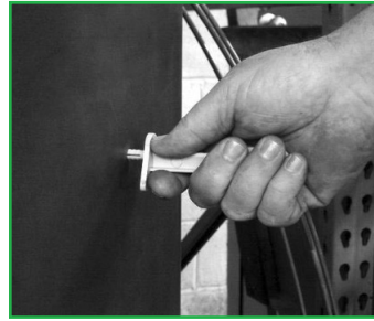
STEP 2: Insert locking mechanism into drilled hole.
