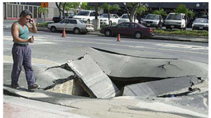
Excessive leaking can lead to pavement collapse when the integrity of the soil is compromised.
