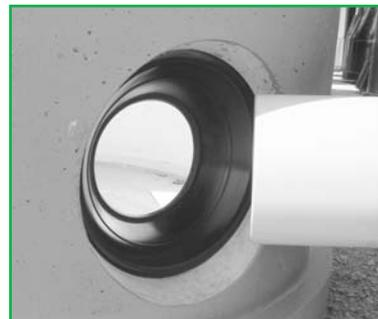
**INSIDE Z-LOK CONNECTOR INSTALLATION**
