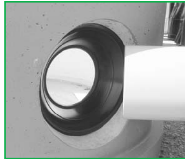
INSIDE Z-LOK CONNECTOR INSTALLATION
