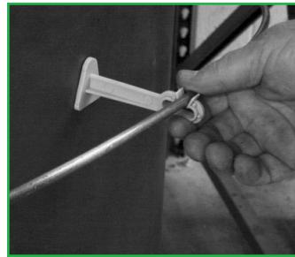
STEP 3: Align Hoop in Cradle all the way around.
