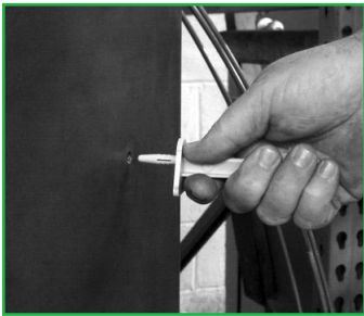
STEP 1: Align locking mechanism into drilled hole.
