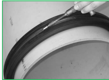
(Fig. 1) Tightening down one piece spliced WATER-STOP with torque wrench prior to grouting.
